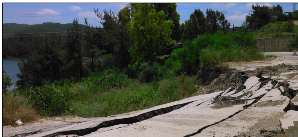
Figure 3.7: Damage to the road network caused by a landslide near Balloran in 2019.
